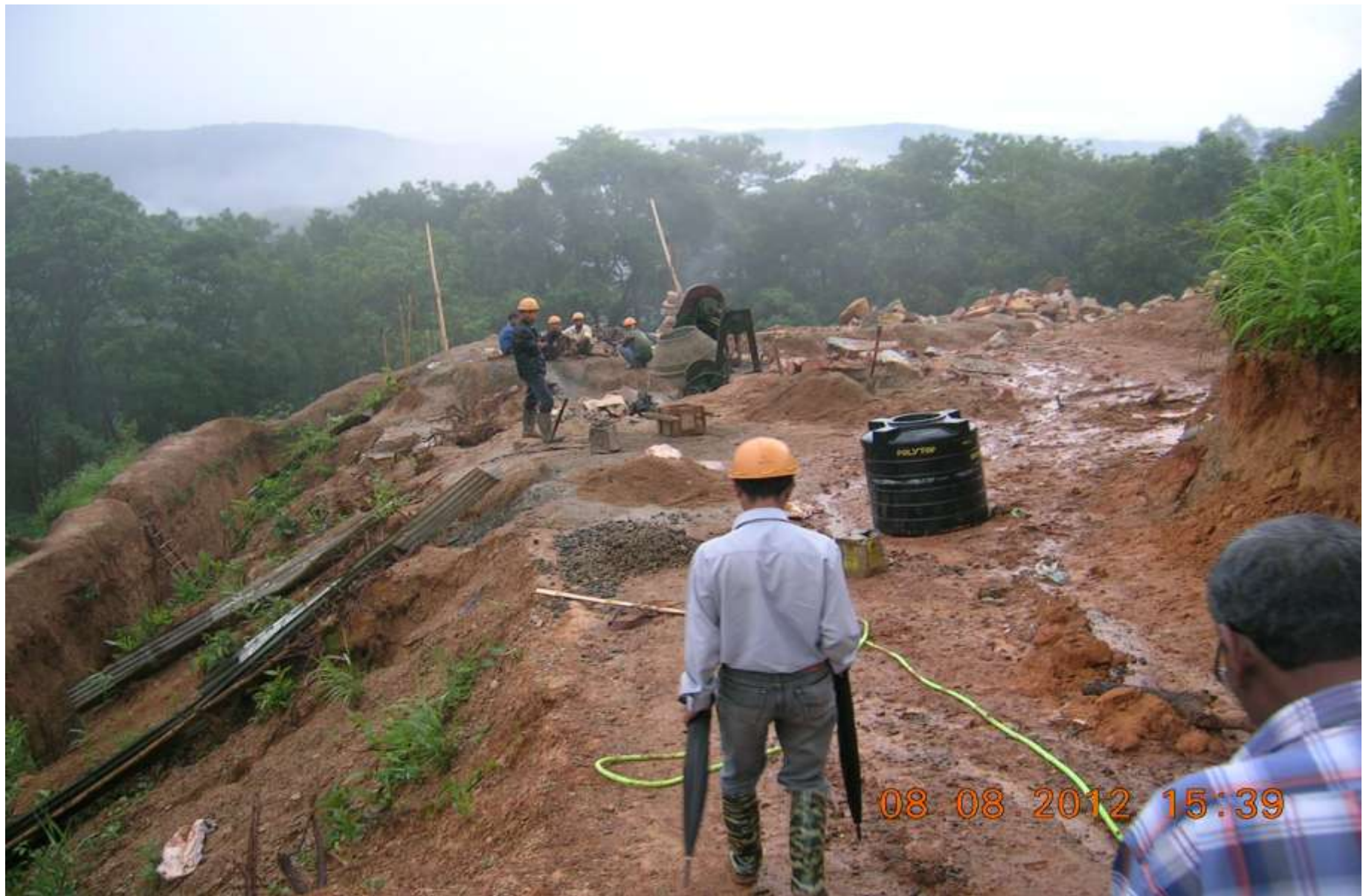
Construction of SLF in progress
