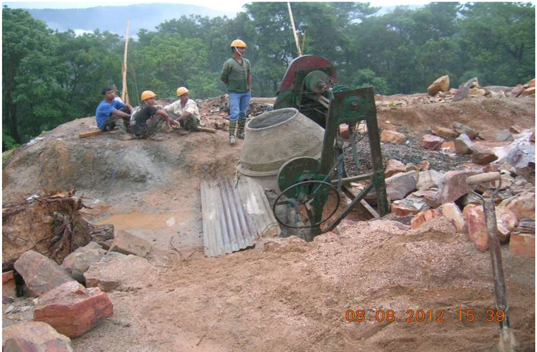
Construction of Retaining Walls under progress 8
