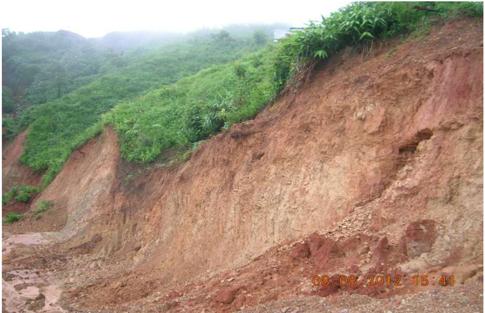
Earthwork and Retaining wall work in progress 6
