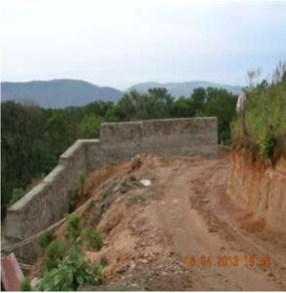
Stone Masonary retaining Wall
