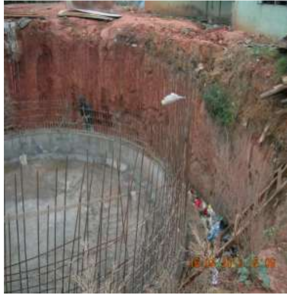
Construction of water reservoir
