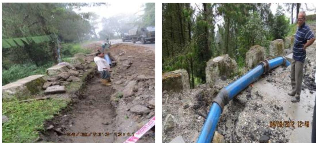
The pipework includes building of about 7 Break Pressure Tanks (BPTs). Of these 2 are under construction. We understand there is some difficulty in obtaining land for construction of the BPTs. SIPMIU should take advance action to finalize the location of BPT tanks and arrange land. In case of difficulties, they may consider substituting the BPTs with pressure reducing valves. The picture below shows construction of break pressure tanks.
