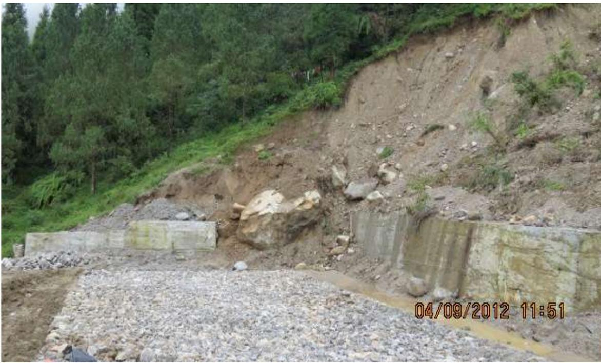
**Soling of the reservoir floor completed, ready for casting PCC**
