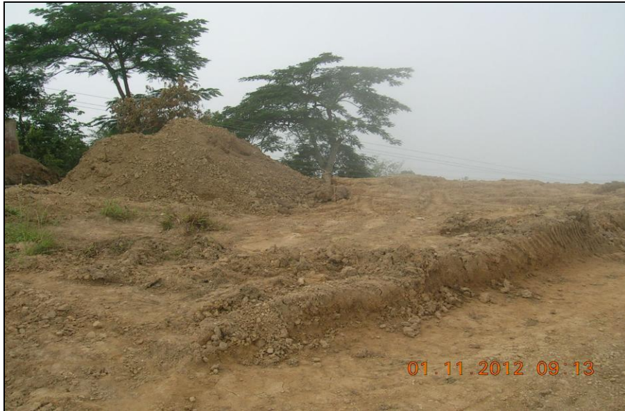
Excavation Work in hand for preparing the base of the tank
