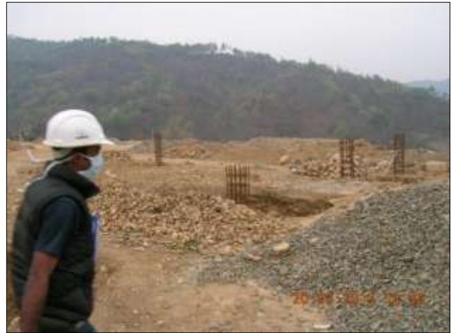
Foundation for compost plant
